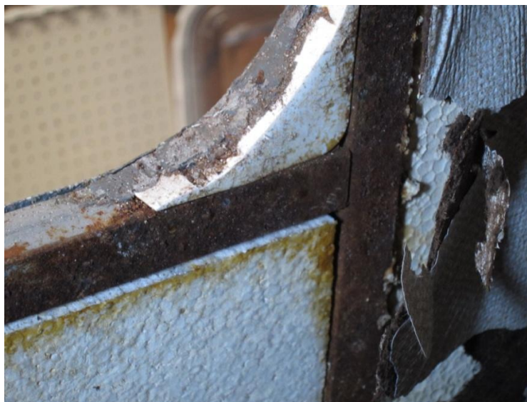
Insulation and metal framing of an older caravan
